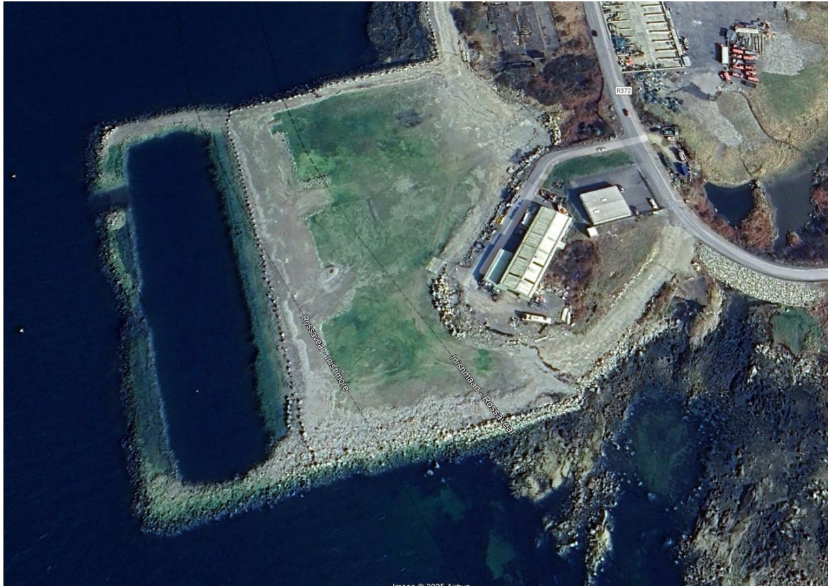
Figure 13-9: Development site in March 2025 (Source: Google Earth Pro)
